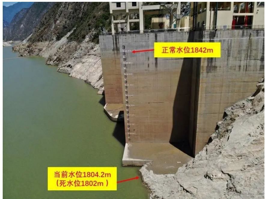
Figure 3: Houziyan Hydropower Station Water Level Comparison
